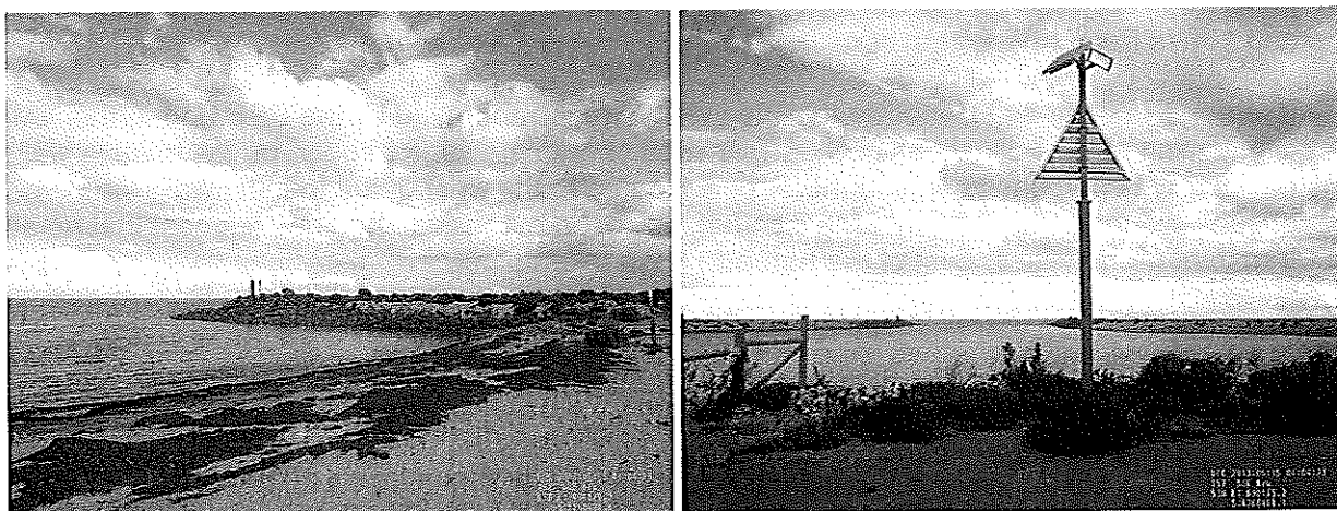
Figure 16 Eastern Training Wall and Ferry Harbour
